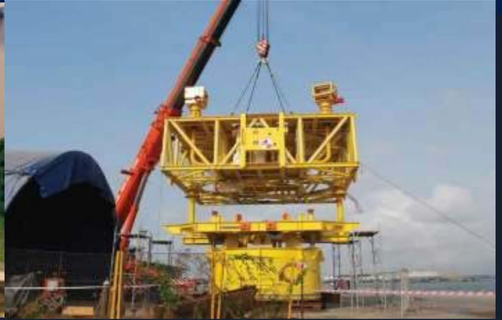
**Subsea Pipeline End Manifold
